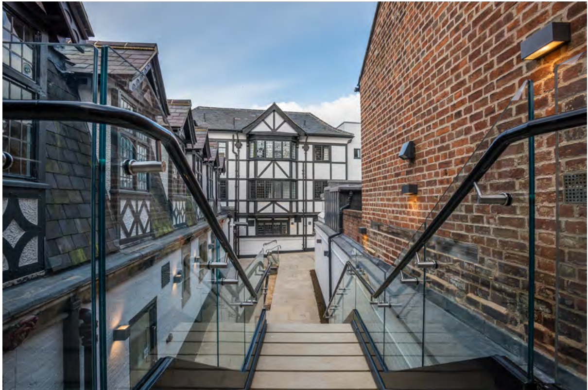
A new walkway through the rear of the building
